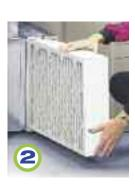
The filter cabinet comes standard with a MERV 8 filter. For customers who desire a higher level of filtration efficiency, a MERV 11 filter is also available.
